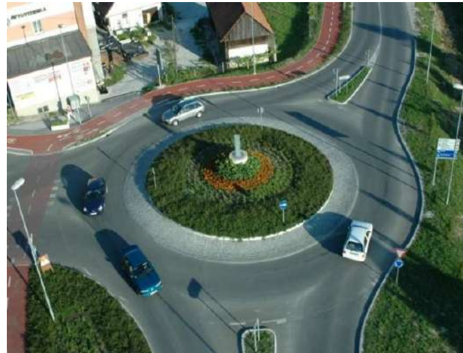
Two lane roundabout on Pesnica – Slivnica motorway
